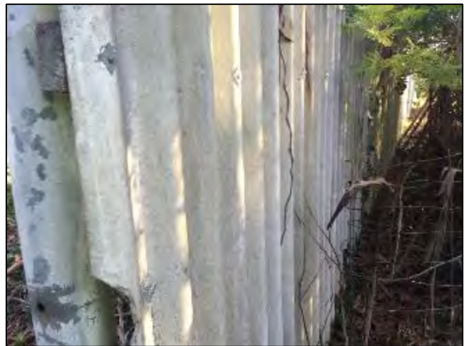
Plate 16 – ACM clad fence in the central portion of the site in moderate condition.
