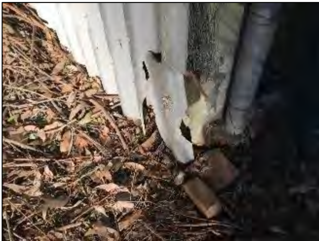
Plate 17 – ACM clad fence in the central portion of the site in moderate condition.
