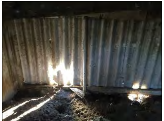
Plate 46 – Damaged ACM cladding in the rear kennels.
