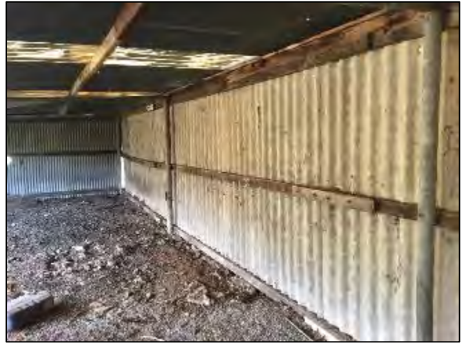
Plate 44 –ACM cladding in the rear shed.
