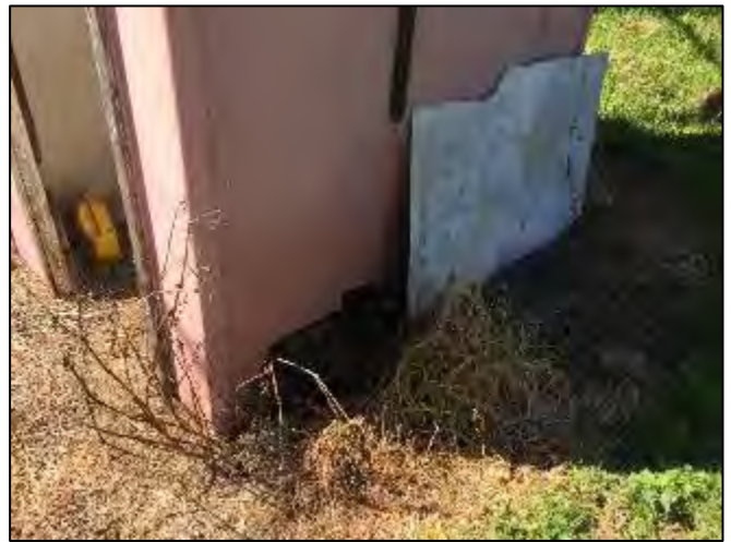
Plate 10 – Damaged ACM cladding on the outhouse.
