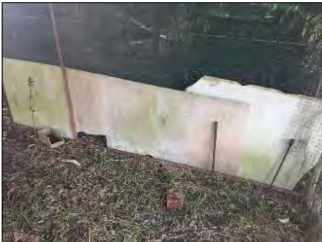
Plate 45 – ACM sheet used to patch fencing in the kennels.
